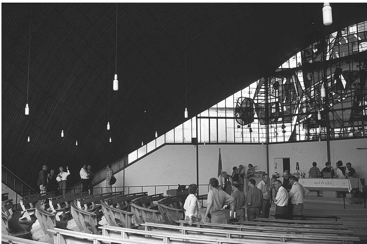
Members of SAHGB studying the concrete hyperbolic paraboloid roof of Sam Scorer's St John, Lincoln (1962-3), during the 1999 Conference. (photograph by Frank Salmon)
